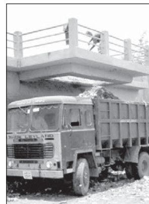
This transfer station has split levels for direct transfer of waste from a small vehicle to a large vehicle.
